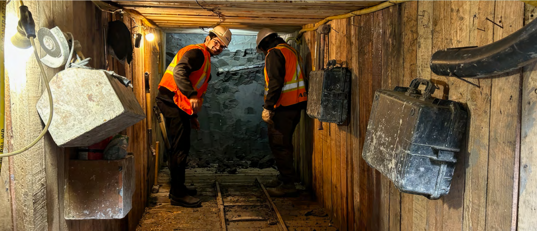
Enwave team members in a hand-mined tunnel connecting a customer to the district
