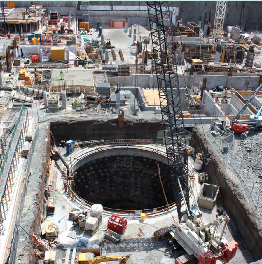
The Well storage tank under construction
